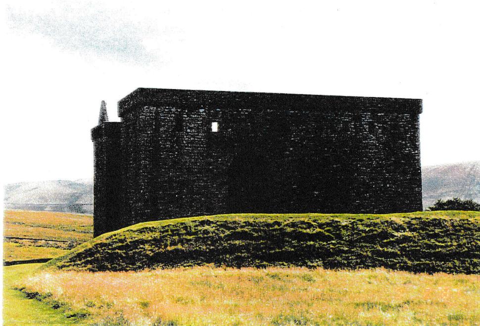
Hermitage Castle, Liddisdale Built in the Thirteenth Century, by the end of the Eighteenth Century, it had fallen into complete disrepair.
